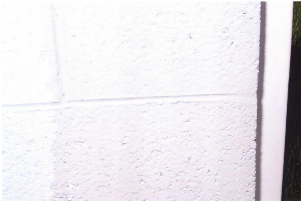
9. Close-up of wall after rinsing the graffiti removed area with water. Note the complete removal of the graffiti with no staining, ghosting or shadowing.
