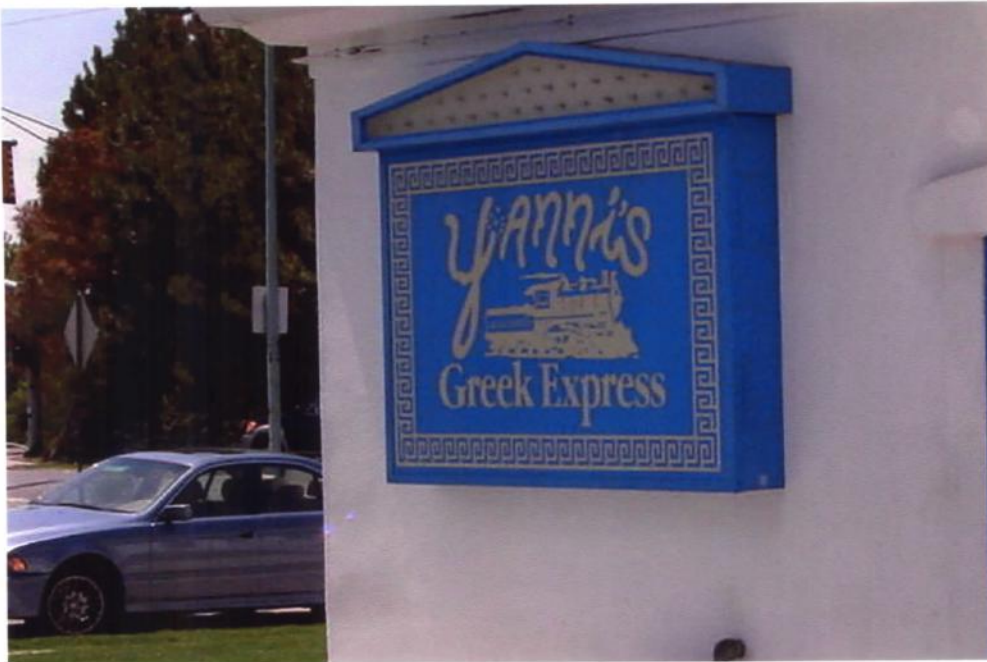
11. Flat, white color coat GSS system applied to sand textured stucco.
