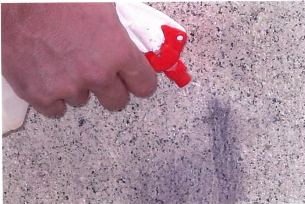
30. Applied graffiti being removed with Erasol.
