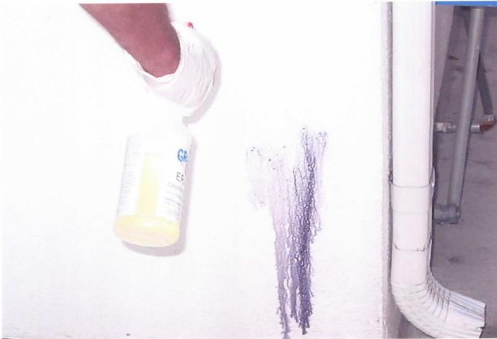
13. View of spray application of Erasol to the graffiti. Note how the graffiti is totally dissolved by the remover.
