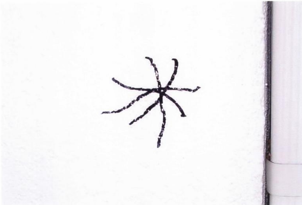
12. Flat, white sand textured stucco wall with black permanent marker type graffiti.
