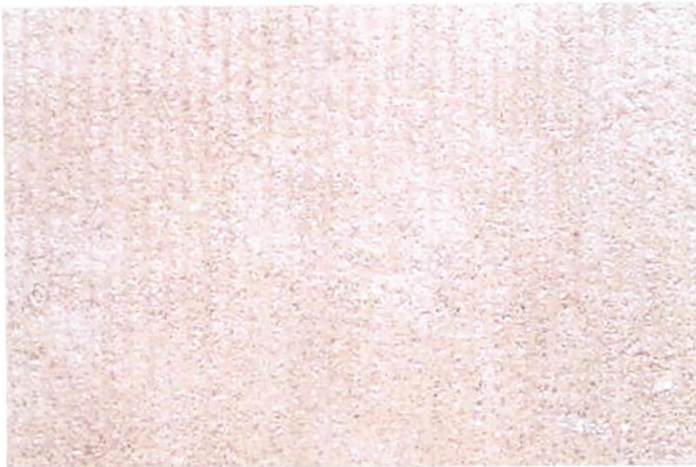
28. Close-up of surface after removal. Note the total lack of any black staining.
