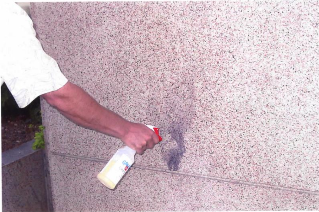
21. Applied graffiti being removed with Erasol.
