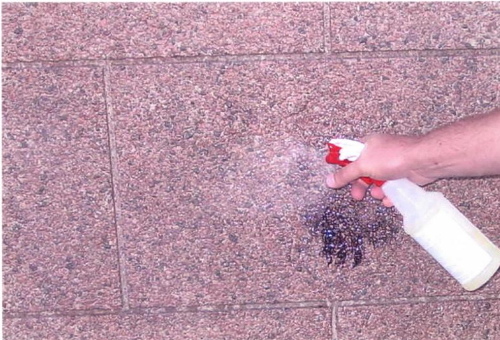
16. Applied graffiti being removed with Erasol.
