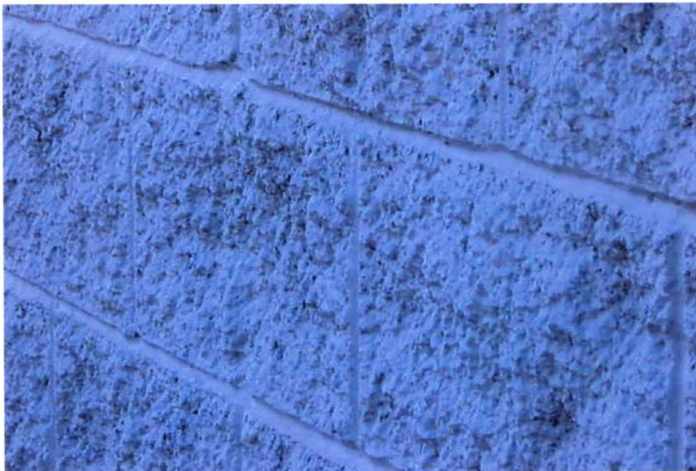
4. A more porous split-face block surface at the Palo Verde High School that has been treated with a base coat system containing a greater amount of filler.
