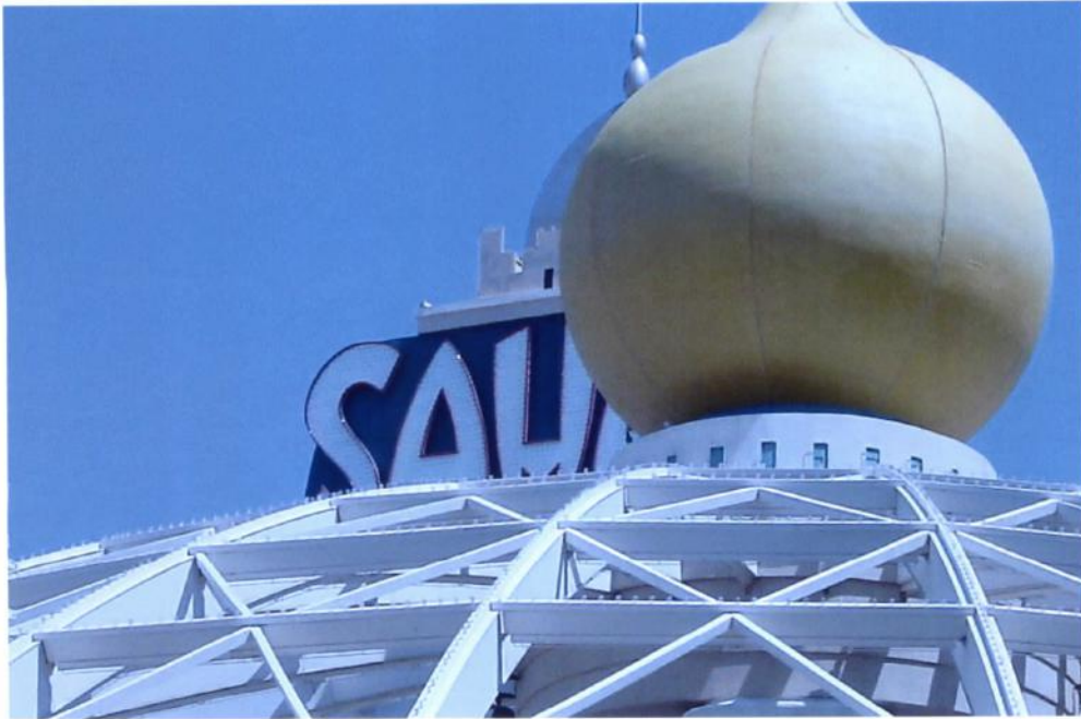
1. Foam-skinned dome at Sahara protected with flat color coat system. Note uniformity of appearance after 6 years of exposure.
