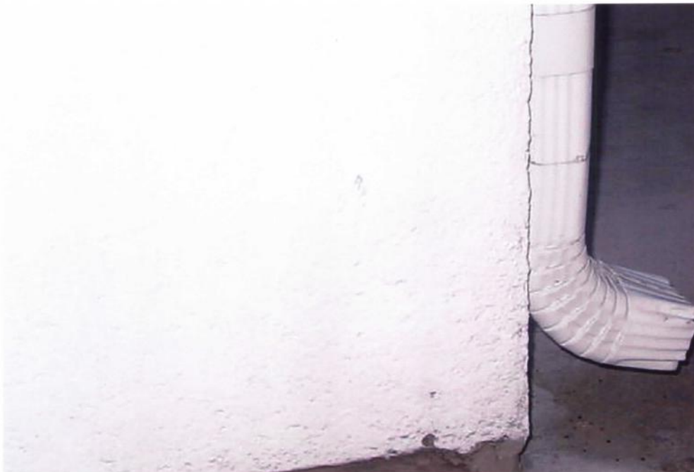
14. View of the stucco wall after removal of graffiti with Erasol. Note the total removal of the black markings with no apparent change to the white color coat.
