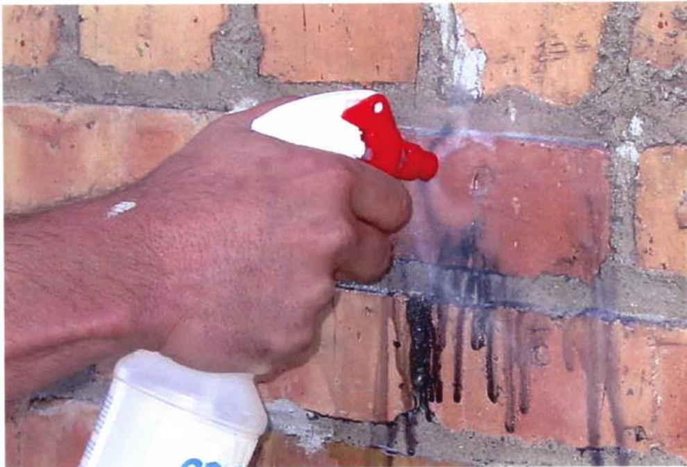
24. Applied graffiti being removed with Erasol.
