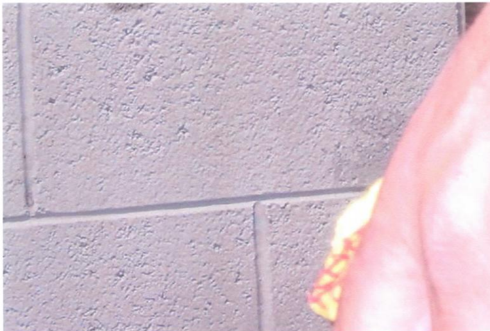
10. Close-up view of wall after drying. Note that the color coat has been virtually unaffected by the Erasol - there is no change in color or gloss when compared to the surrounding areas of wall after graffiti removal.
