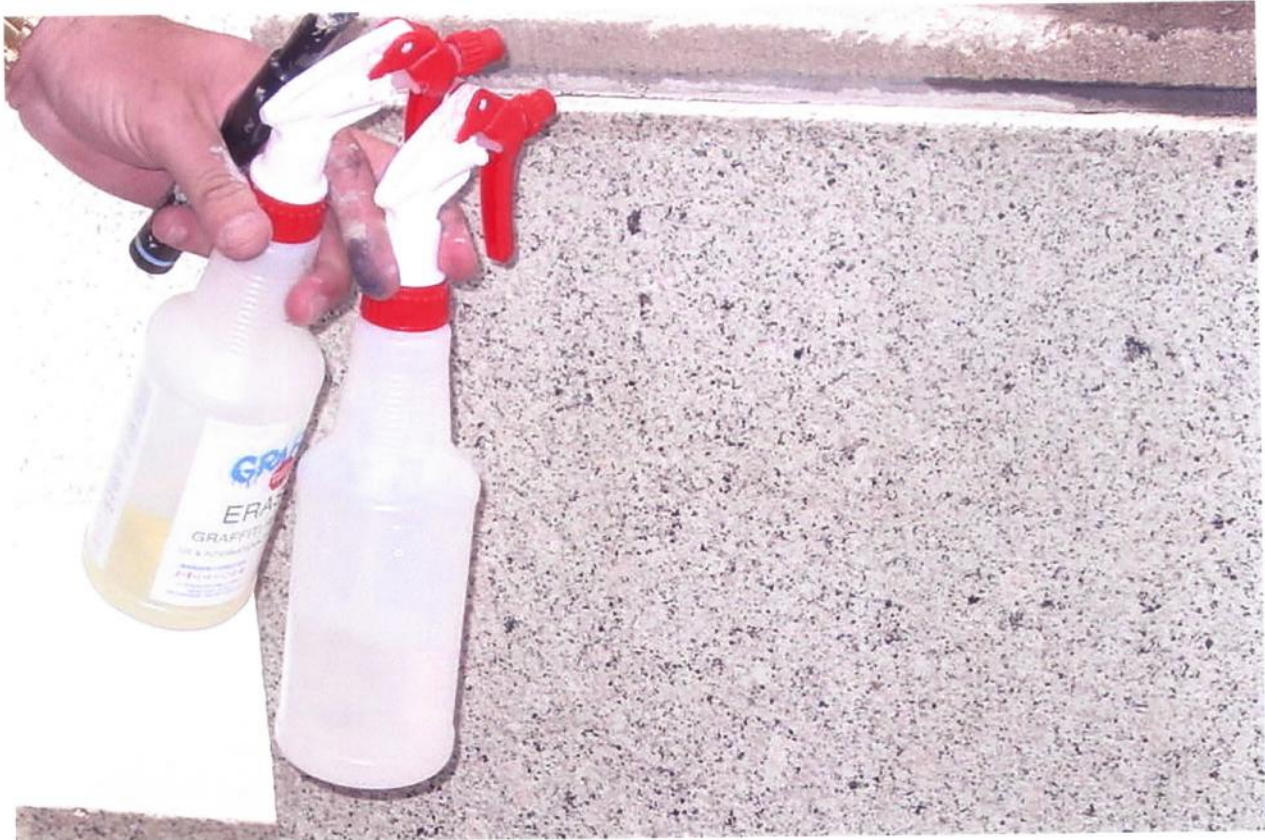
31. Close-up of surface after removal. Note the total lack of any black staining.
