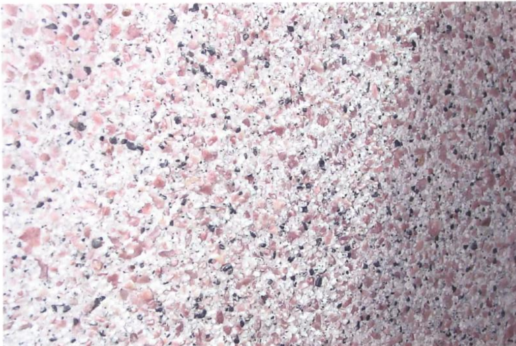
22. Close-up of surface after removal. Note the total lack of any black staining.
